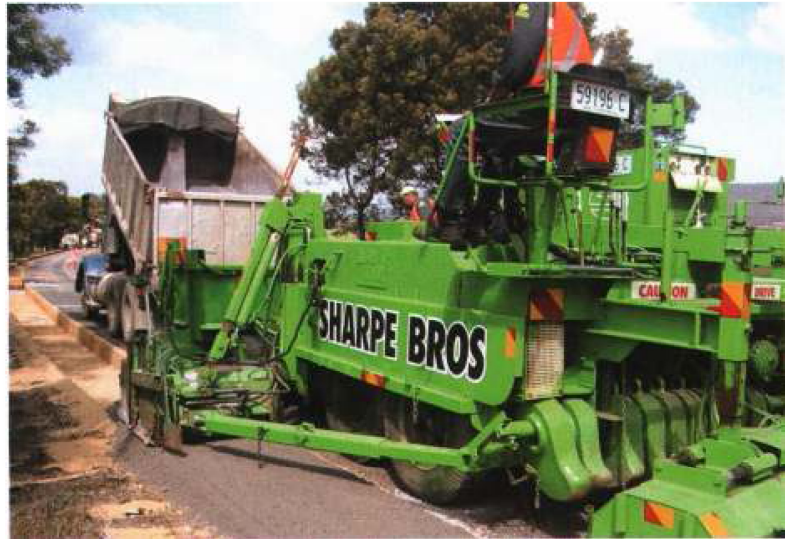
The Sidewinder machine is designed to fix pavement edge drop-offs
